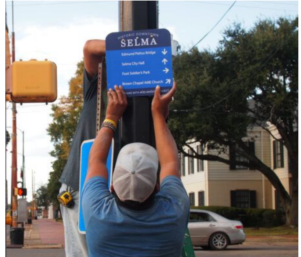
Installing wayfinding signs in Selma, AL
